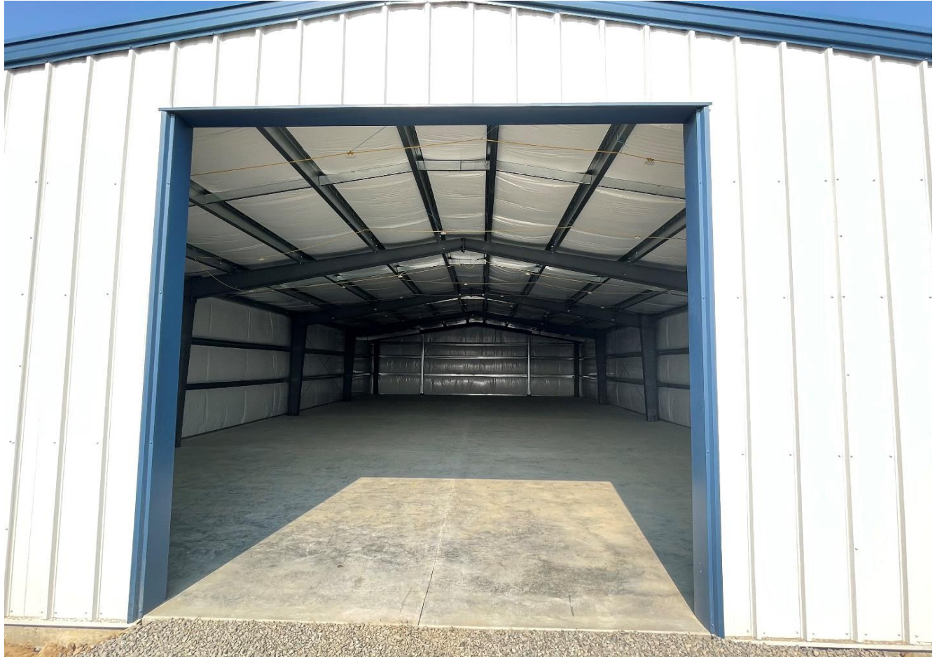
PHOTO OF FINISHED WORK. FRANCHESKA'S STORAGE INSTALLATIONS LLC.
