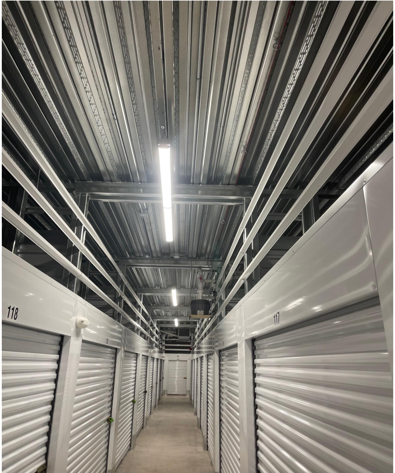
PHOTO OF FINISHED WORK. FRANCHESKA'S STORAGE INSTALLATIONS LLC.
