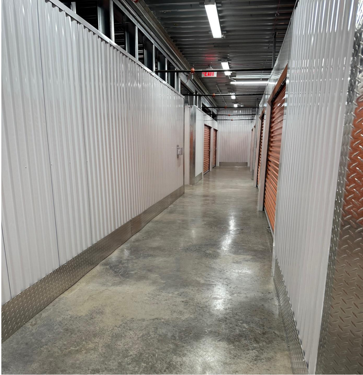
PHOTO OF FINISHED WORK. FRANCHESKA'S STORAGE INSTALLATIONS LLC.
