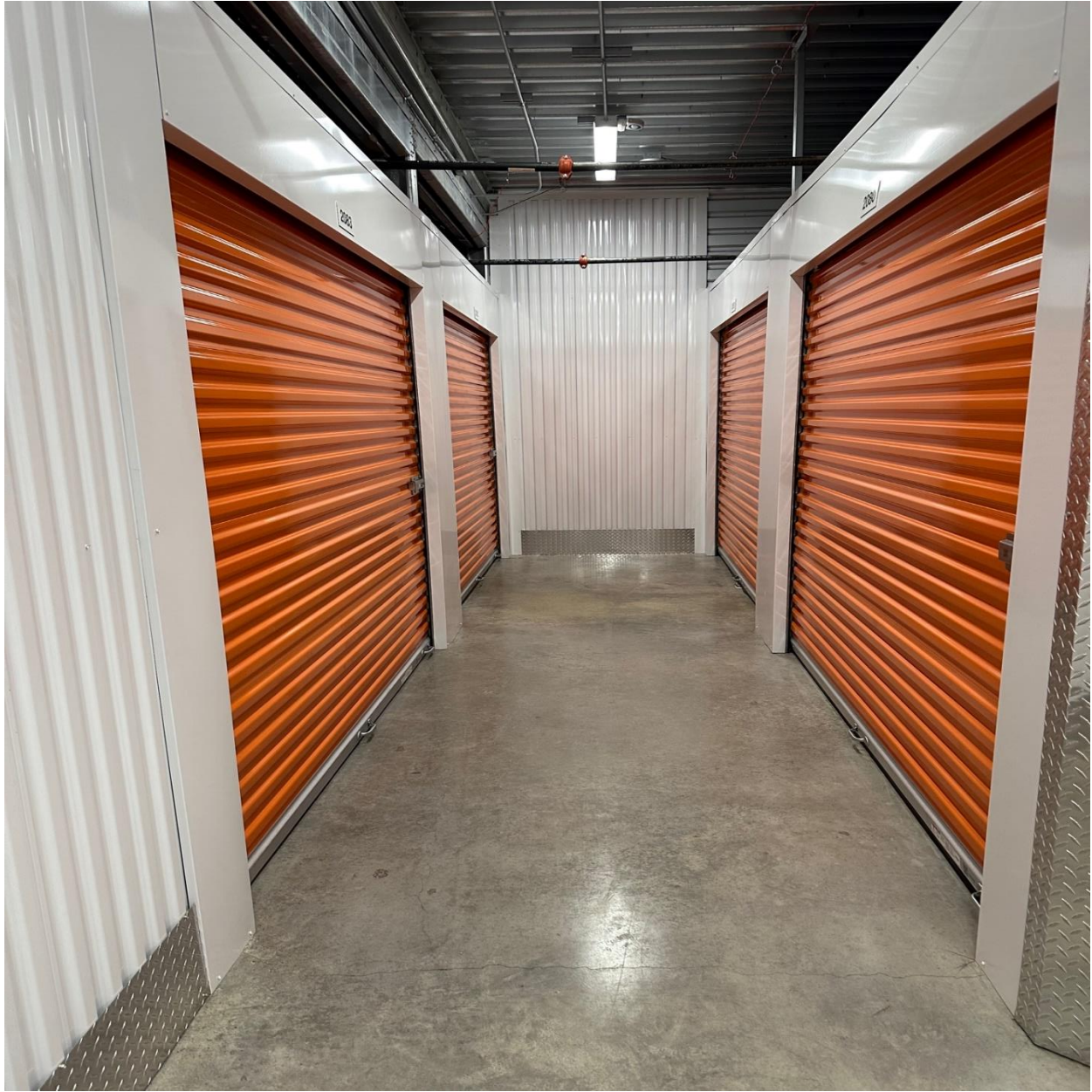
PHOTO OF FINISHED WORK. FRANCHESKA'S STORAGE INSTALLATIONS LLC.
