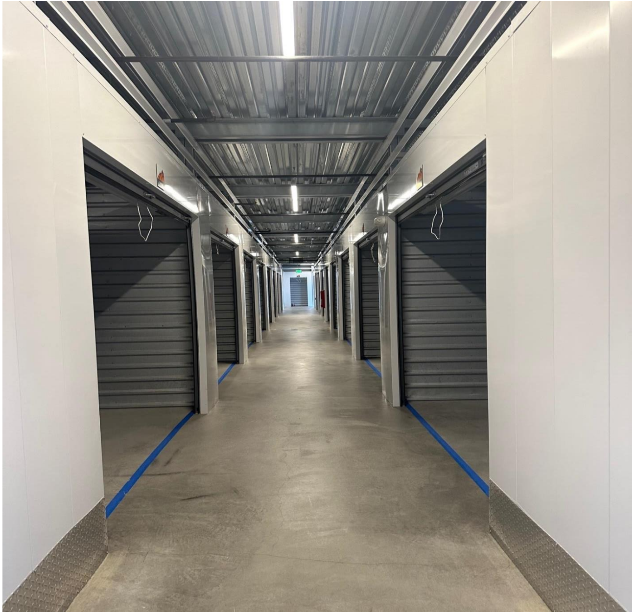
PHOTO OF FINISHED WORK. FRANCHESKA'S STORAGE INSTALLATIONS LLC.
